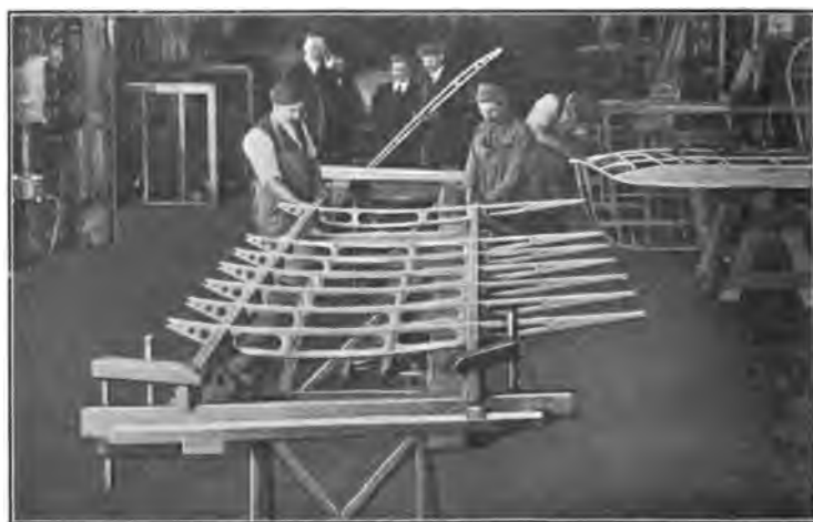
FIG. 131.—Assembling wing with spars.
